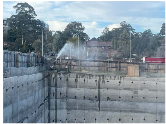
Photos 19 & 20: Excavation of the basement structure was ongoing. Water cannons were in place to reduce dust
