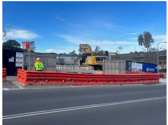
Photos 15 & 16: A work zone had been established to load-out VENM on De Clambe Drive. Signage and traffic control was in place as required.
