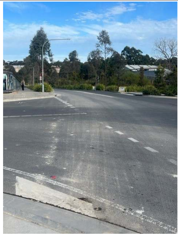
Photos 17 & 18: Minor tracking was observed from the work zone / VENM load-out zone onto De Clambe Drive
