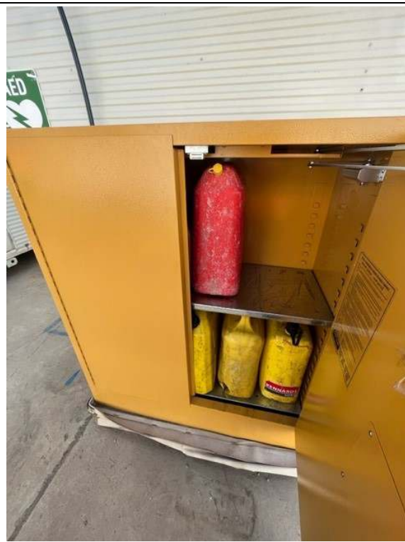
Photos 6 & 7: Jerry cans of ULP and diesel were stored inside a purpose-built container. The container required labelling in accordance with the GHS
