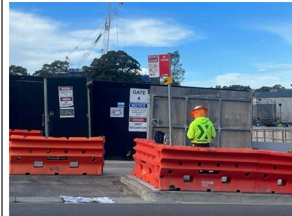
Photos 15 & 16: A work zone had been established to load-out VENM on De Clambe Drive. Signage and traffic control was in place as required.
