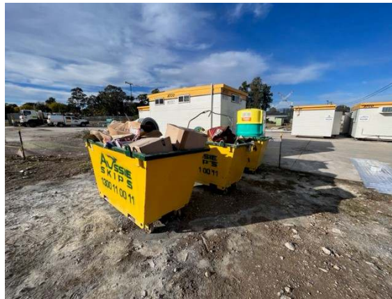
Photo 3: Skips containing construction waste. Empty oil and fuel containers are removed by the surface mining company for appropriate disposal
