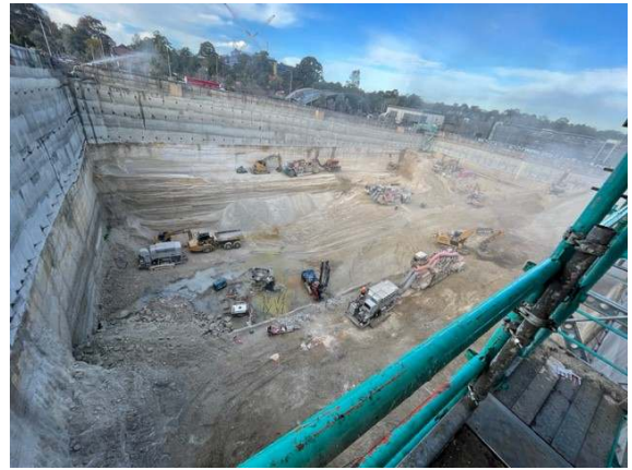
Photos 19 & 20: Excavation of the basement structure was ongoing. Water cannons were in place to reduce dust
